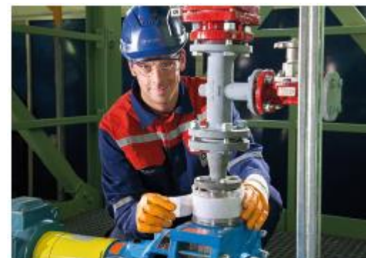
↑ Assembly of the safety tape flange connection
